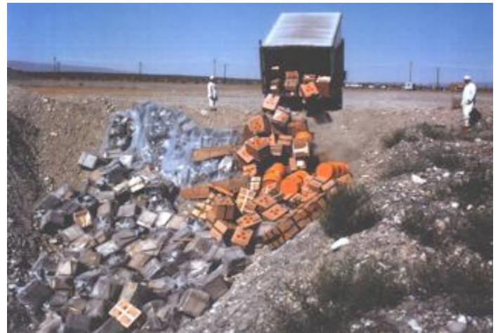
Radioactive waste being dumped into unlined trenches
